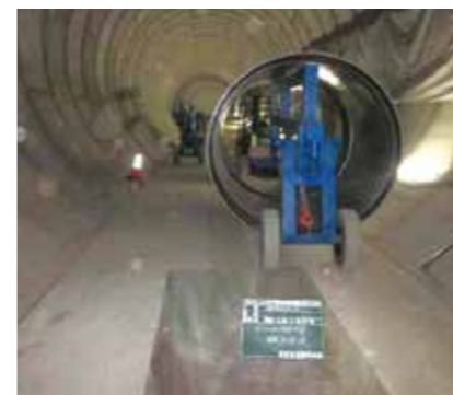
FRPM管運搬
