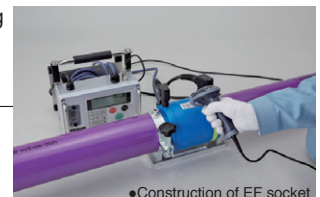
●Construction of EF socket
