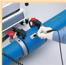
Constructing EF socket
