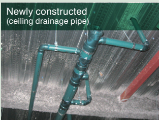
Newly constructed (ceiling drainage pipe)
