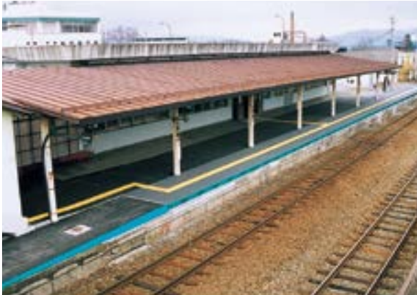
Platform raising work
