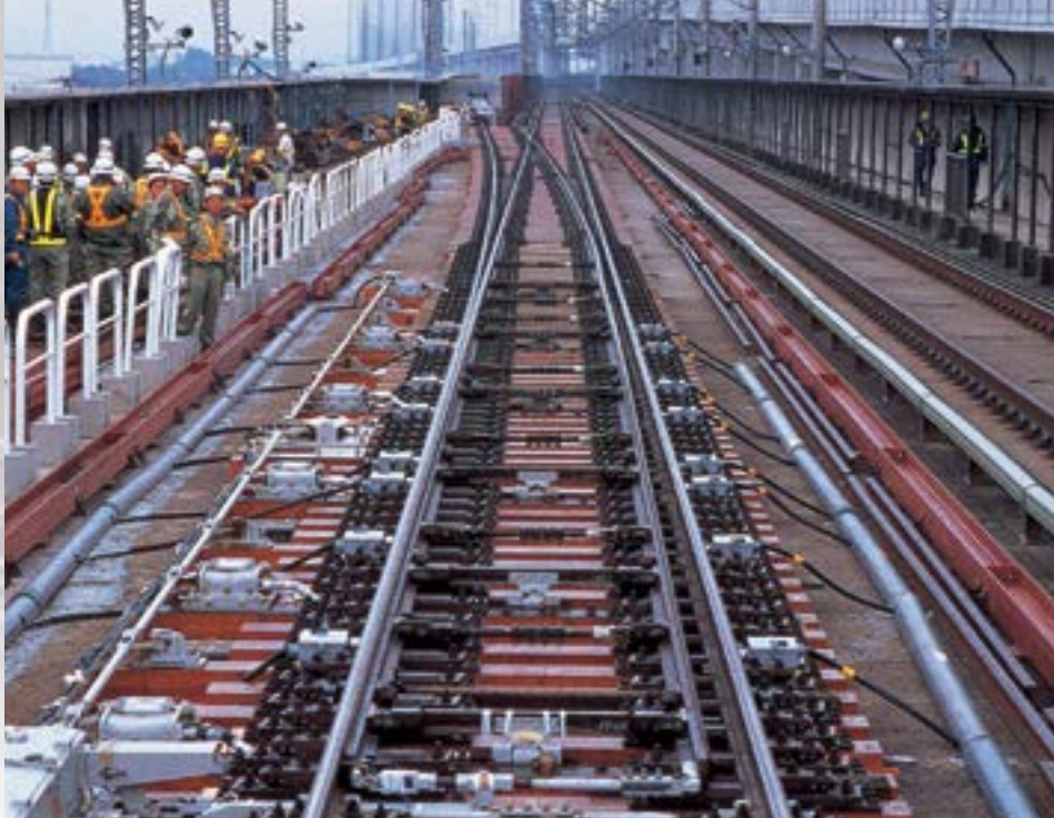
Takasaki #38 switch sleeper, largest in Japan (Hokuriku Shinkansen)
