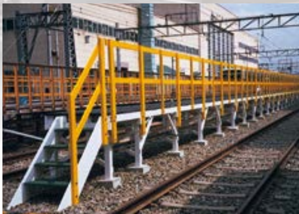
Deck of car washing area
