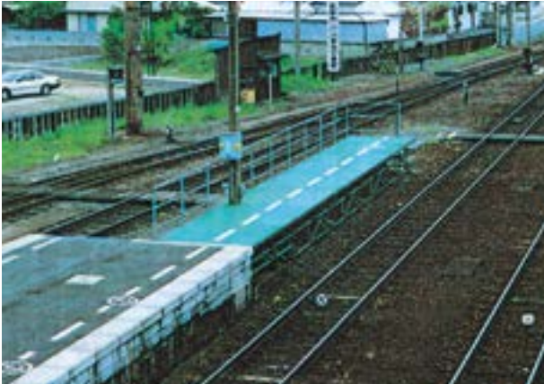
Platform extension work
