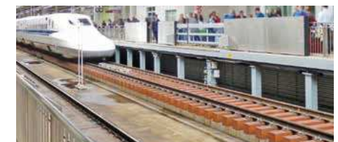
Track built on synthetic railway sleepers for Line No. 27 at Shin-Osaka Station
